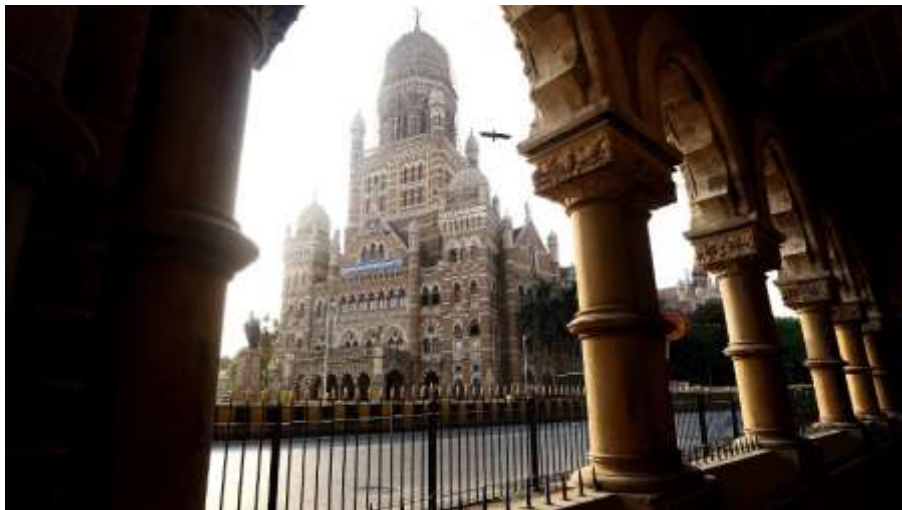
The Brihanmumbai Municipal Corporation (BMC) building in Mumbai | ANI
